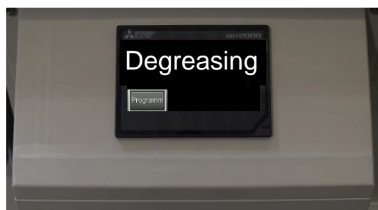
Control panel for process control (Example: degreasing)
