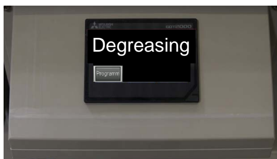
Control panel for process control (Example: degreasing)
