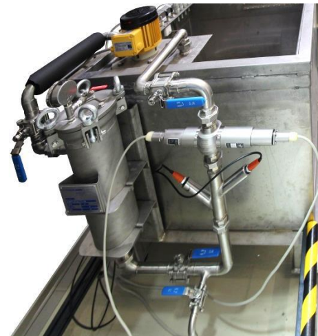
Filter bag unit and sensors for monitoring the plating bath
