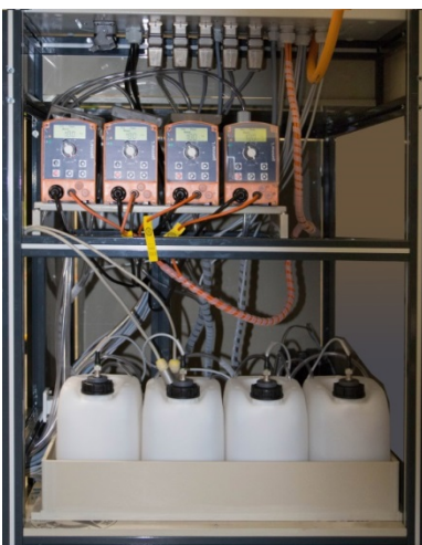
PRS 内视图：计量泵和镀槽化学剂的贮池 Innr view of PRS: Dosing pumps and reservoirs for regulation chemicals for plating bath
