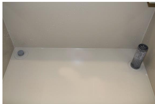
冲洗槽内视图 Inside view of rinsing tank
